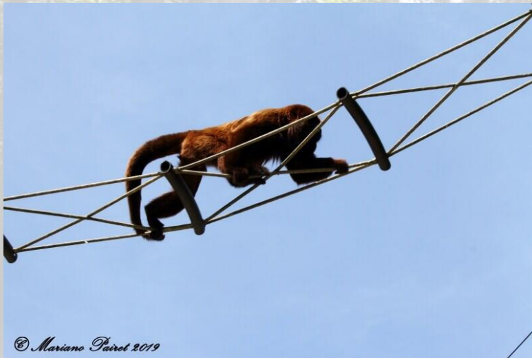
Figure 1. Construction of rope overpass with four 12 mm ropes interlaced and rubber hose to form ladder steps. Author: Elisandro Oliveira dos Santos.
